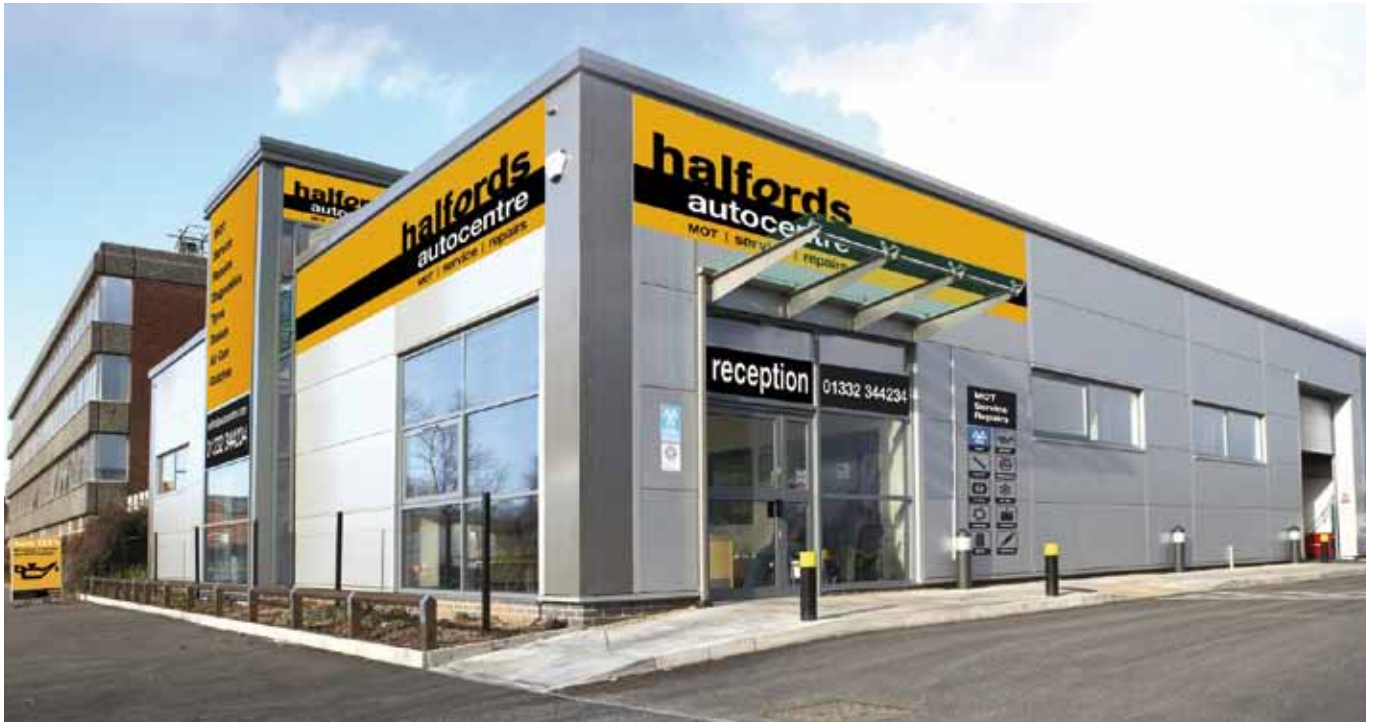
Pictured: Unit 1, Saxondale Park, London Road, Derby.
