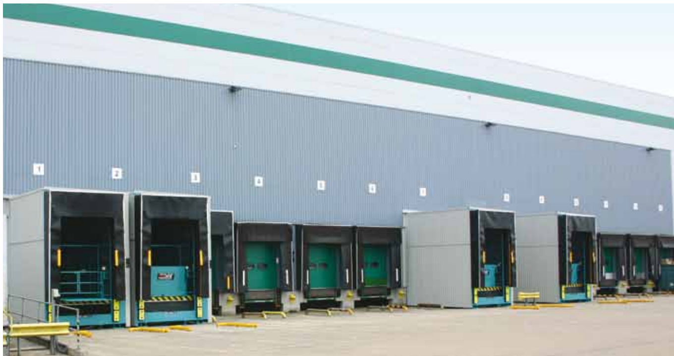
Pictured: Loading bays, new Coventry DC.
